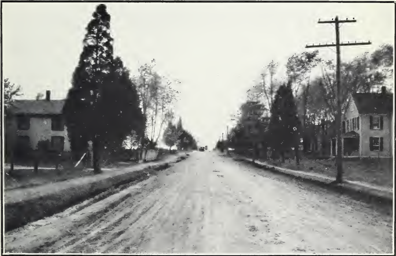
FIG. 2.—CLAY-GRAVEL ROAD IN VIRGINIA MAINTAINED BY A ROAD DRAG.
